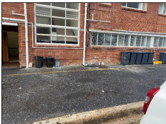
Figure 11. Open door providing access to the kitchen and unsecured waste bins at Job Maseko Barracks.
